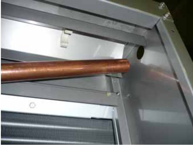
Figure 13: Installation of Copper Waterfeed Pipe
