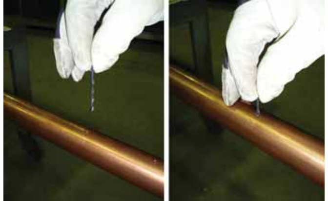
Figure 10: Clean Spraying Holes
