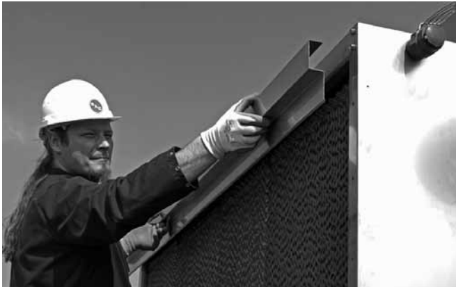
Figure 19: Remove Top Plate
