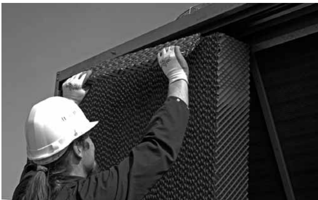
Figure 20: Removal Water Distribution Pads
