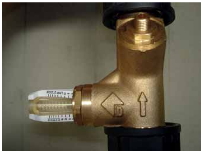
Figure 3: Water Flow Adjustment Screw
