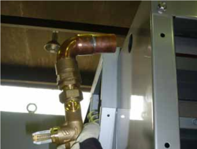
Figure 7: Waterfeed Connection
