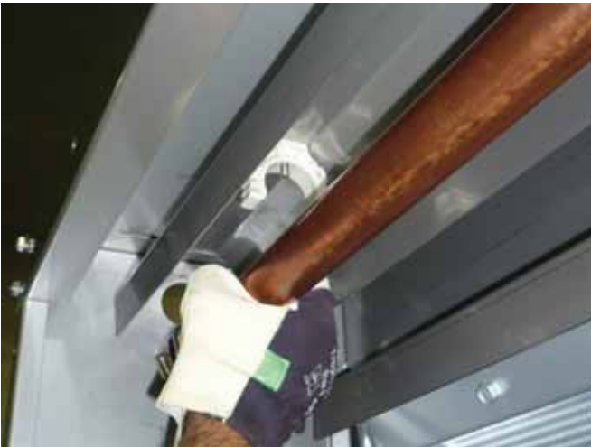
Figure 8: Release Copper Collector from Plastic Holders
