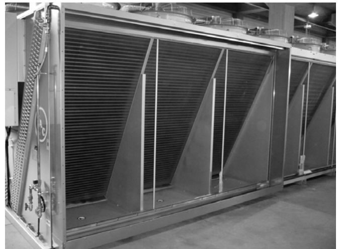
Figure 5: Unit without Pre-cooling Media
