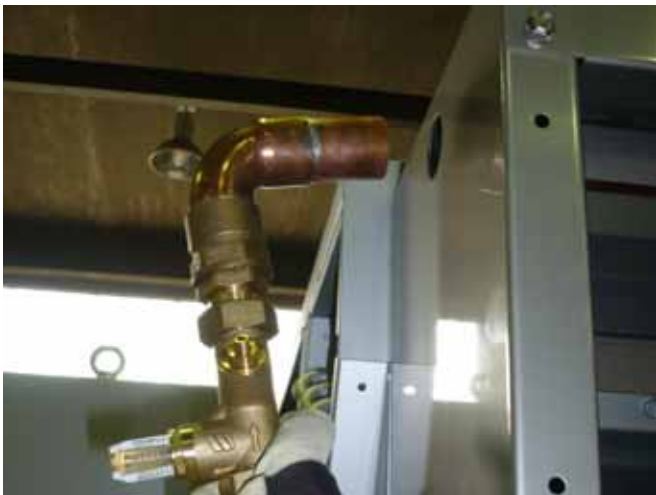
Figure 15: Waterfeed Assembly
