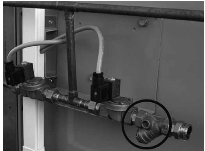
Figure 4: Water Filter
