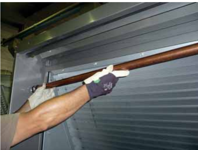
Figure 9: Remove Copper Waterfeed Pipe
