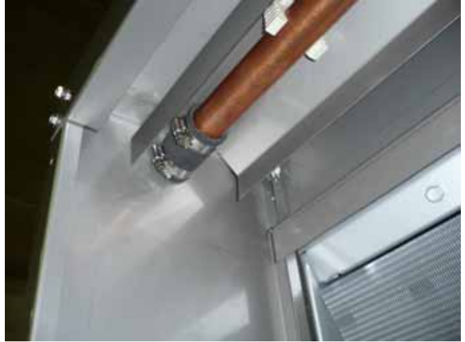
Figure 16: Flexible Sleeve Connection with Sleeve Clamps
