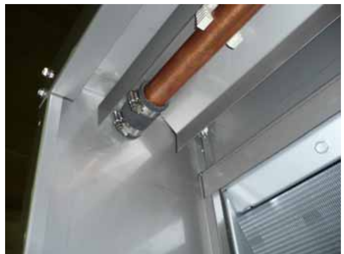
Figure 6: Flexible Sleeve Connection
