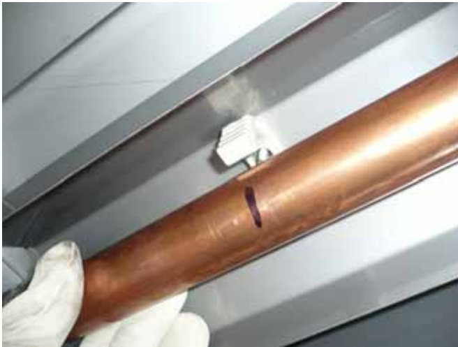
Figure 14: Alignment of Waterfeed Pipe
