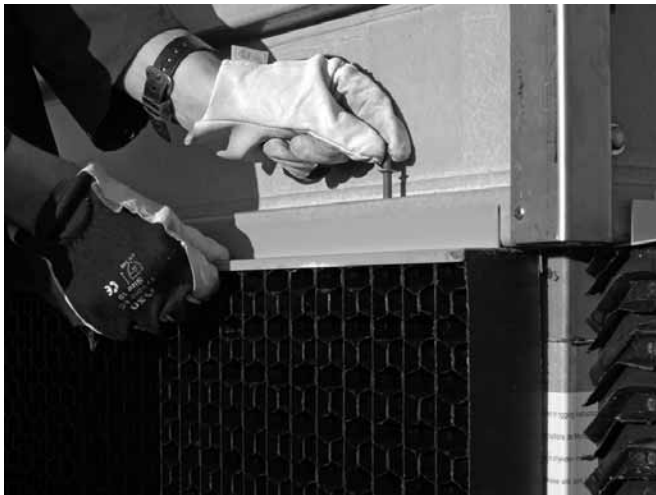
Figure 12: Remove Combined Inlet Shields
