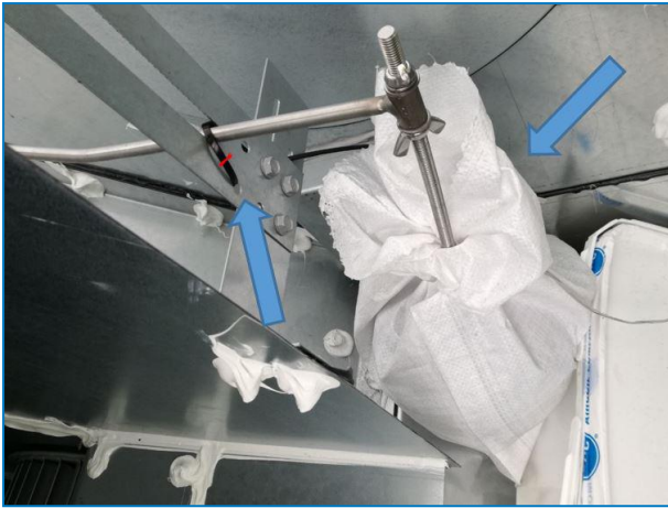
Fixation and wrapping of Float ball
