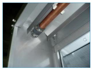
Flexible Sleeve Connection with Sleeve Clamps
