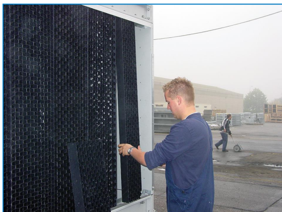
Remove Combined Inlet Shields
