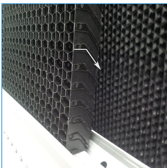
Orientation of the combined inlet shield
