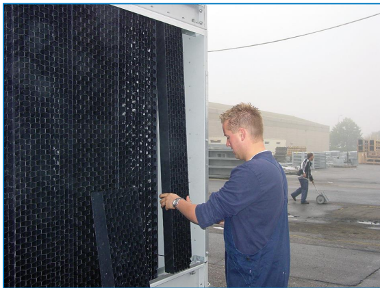
Remove Combined Inlet Shields
