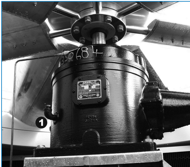
Single Reduction Gear Drive
