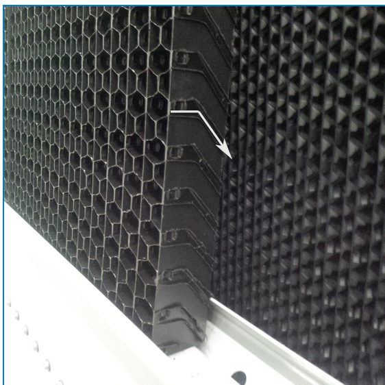
Orientation of the combined inlet shield
