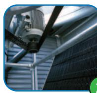
A single low noise axial fan per condenser is installed offering 50 % lower energy consumption versus traditional centrifugal fans.
