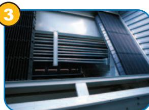
Easy removal of acoustical baffles for inspection and cleaning of the wet deck surface and water basin.
