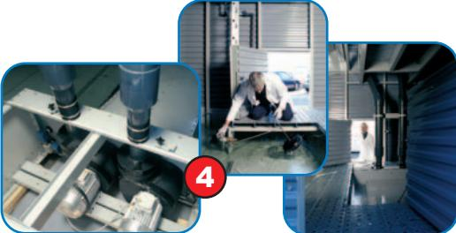
Large hinged access door, internal walkway and spacious plenum for access to mechanical make-up, spray pumps and strainer, as well as other basin accessories. Pumps are located in a separate pump well inside the condenser.
