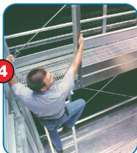
Internal ladder and service platform provides access to fan, motor, drives and coil.
