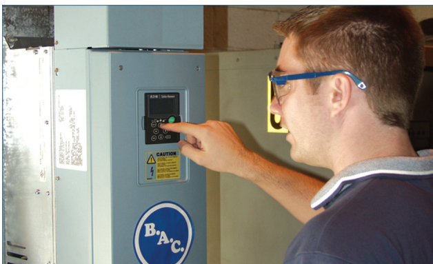
Figure 8: VFD with Integrated Bypass
