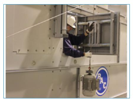
With the motor removal davit, the motor **can easily be lowered from or lifted to** the motor base without the need for extra heavy material of scaffolding.
