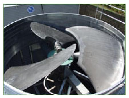
**Quiet and economical kW axial fans** mean FXV-D cooling towers make little sound. To reduce noise still further, choose the **Whisper quiet fan** alternative targeting optimal noise-reduction, with an aluminum hinged-blade design and unique end caps.
