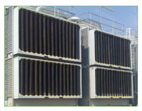
FXV-D closed circuit cooling towers use **quiet and low kW axial fans**, but to reduce noise even further, you can extend your FXV-D with <u>sound attenuation</u>:
