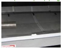
A sump sweeper piping system **increases water circulation and agitation in** the basin and is designed to be used in combination with a filtration system. It does all this:
