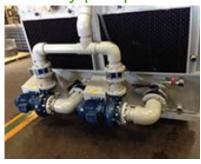
Installing a standby pump guarantees year-round reliable operation – the redundant pump takes over in event of a failure.
