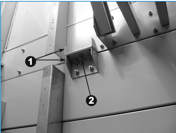
Plenum Section installed on Lower section
