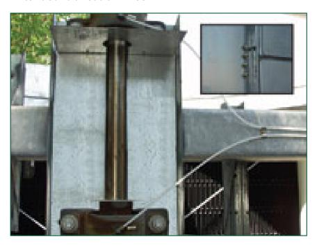
Extended lubrication lines with grease fittings can be used to lubricate fan shaft bearings. The fittings are located inside the plenum area next to the access door.
