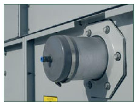
Filling the condensing coil with nitrogen helps **prevent corrosion** during long shipment periods or on-site storage.
