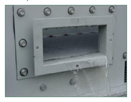
A factory-installed clean out port
