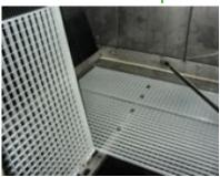
As well as **easy access to internal unit tops**, the installed internal platform also means easier and **safer** inspection and maintenance, in line with **European and South African safety directives**.
