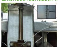
Extended lubrication lines with grease fittings can be used to lubricate fan shaft bearings. The fittings are located inside the plenum area next to the access door.
