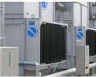
FXVE closed circuit cooling towers use **quiet and low kW axial fans**, but to reduce noise even further, you can extend your FXVE cooling tower with sound attenuation:
