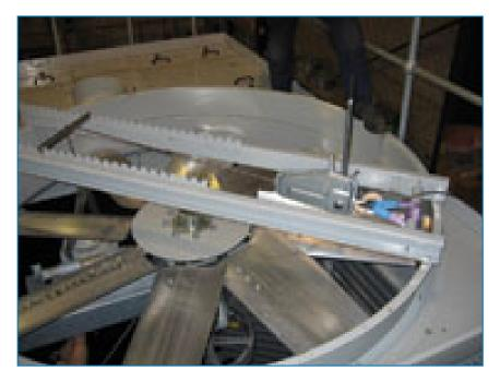
The lightweight mechanical equipment removal system installed helps you **easily remove or install fan motors or gearboxes**.
