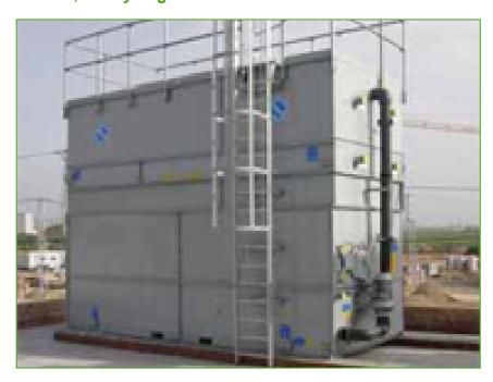
A ladder, safety cage and handrails are all installed for **easy access to the unit top and easier and safer** inspection and maintenance, in line with **European and South African safety standards**. For units equipped with these options, we also recommended installing <u>steel drift eliminators</u>.
