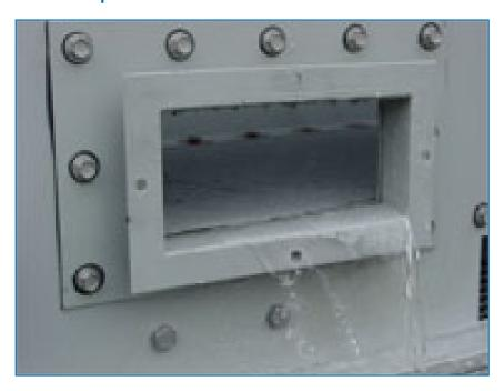
A factory-installed clean out port
