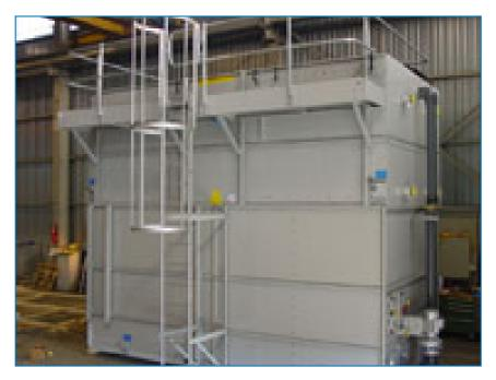
Platforms facilitate **easier** and **safer access** to the **top level** of the unit, making inspection and maintenance easier and in line with European and South African safety standards.
