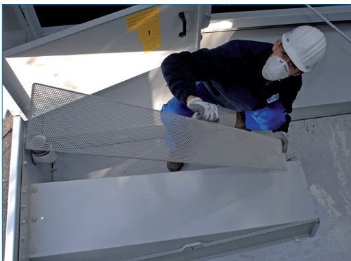
Inspecting Cold Water Basin Strainer
