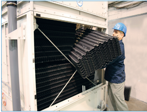
Installing Retrofit Kit
