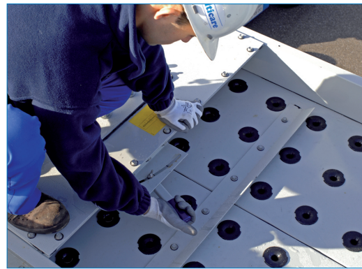
Hot Water Basin with Gravity Water Distribution
