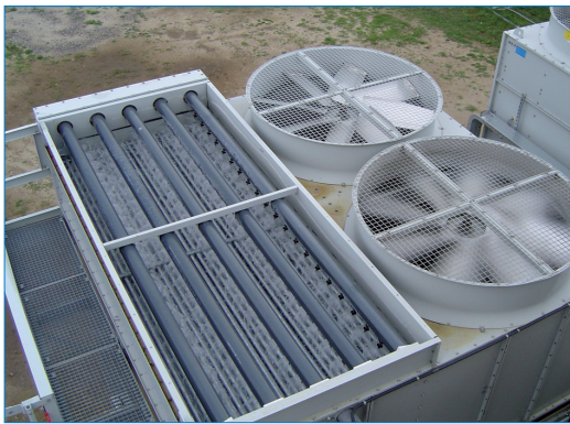
Pressurized Spray Water Distribution
