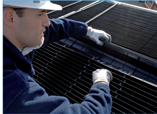
Inspecting Drift Eliminator
