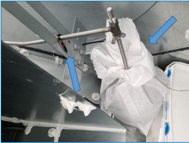
Fixation and wrapping of Float ball
